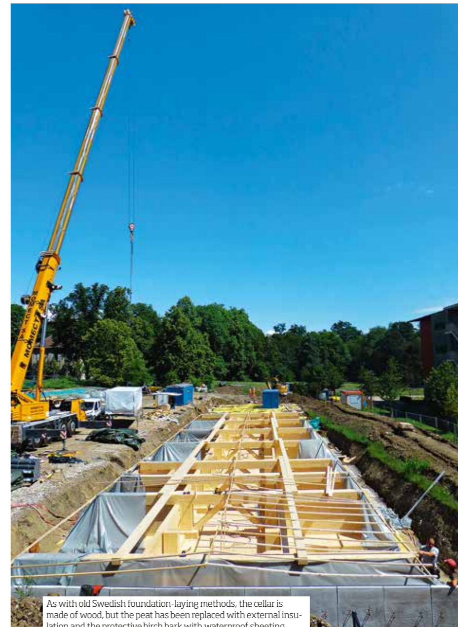
The foundations tend to account for a large part of a building's climate impact, but with debarked larch trees as piles, the footprint can be significantly reduced.
