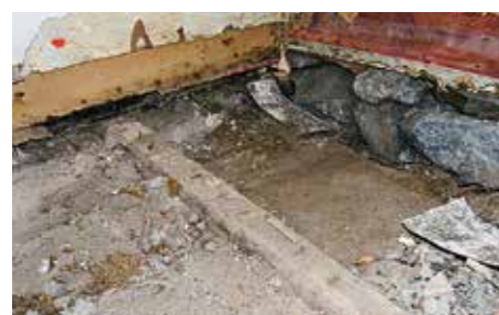
Precursor to the crawl space, a »mullbänk« from an old timber house.
