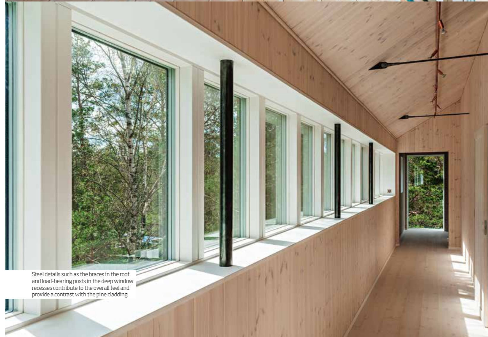
The interior is also defined by natural materials. The floor of tapered pine boards gives a light and welcoming feel that reflects the greenery outside.
