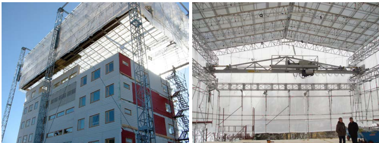
Figure 8.14: a) Movable tent over the whole building. Älvsbacka Strand, Skellefteå, Martinsons Byggsystem, Lindbäcks Bygg AB and White Arkitekter AB (Photo: Anders Björnfot). b) Movable tent from the inside with integrated travelling crane (Photo: Anders Gustafsson).
