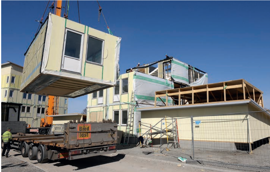
Figure 8.7: Assembly of modular element, Lindbäcks (2013).
